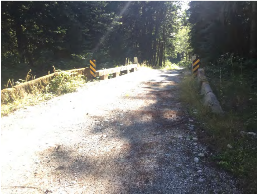
Right Approach Facing Bridge
