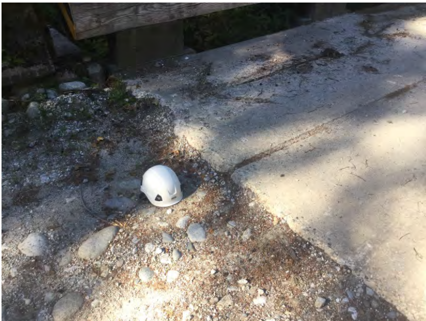
Typical Grade Differential at End of Deck
