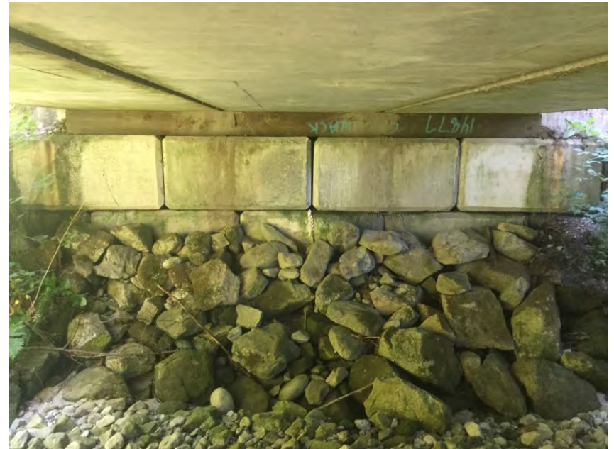
Left Bank Abutment
