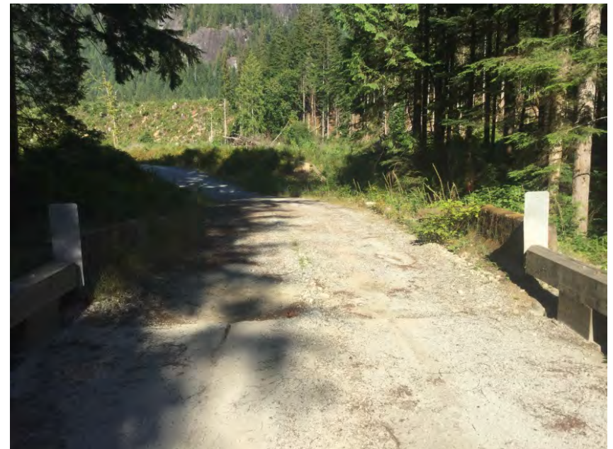
Right Approach Facing Away From Bridge
