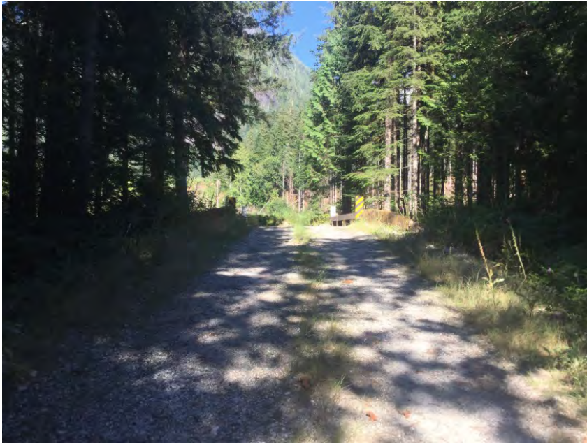
Left Approach Facing Bridge
