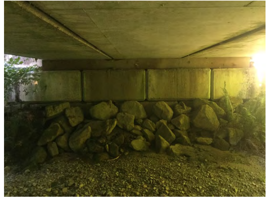
Right Bank Abutment
