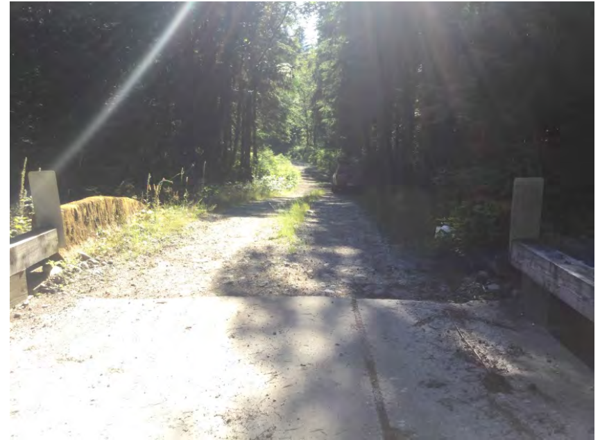
Left Approach Facing Away From Bridge
